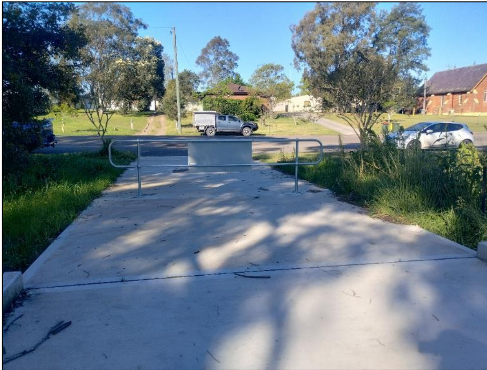
ABOVE: View east toward Grey Street
